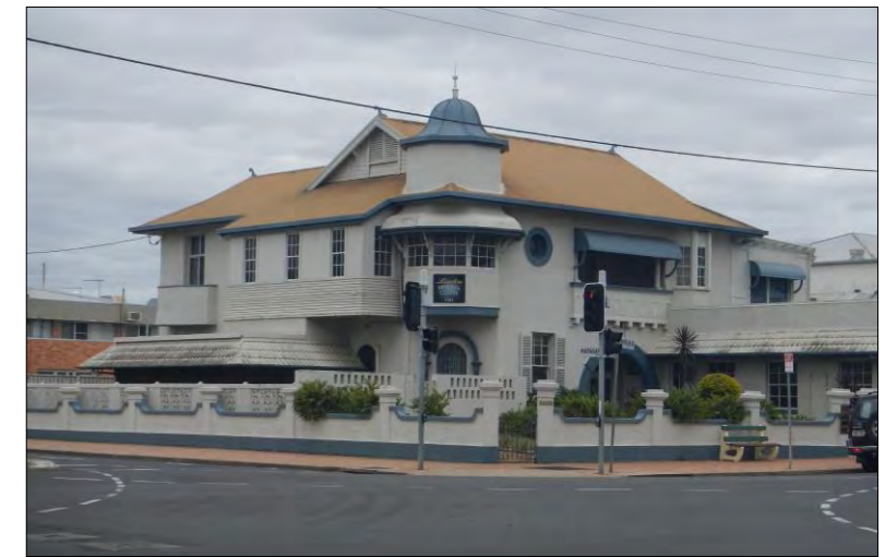
View to original entrance from corner of Woongarra and Barolin Streets.
